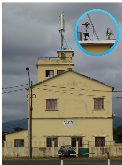
Figure 5. A picture of the STP Instituto Nacional de Meteorologia (INM), with an inset of the Pandora and AERONET instruments temporarily installed on the roof-top. Photo credit: James Podolske.
