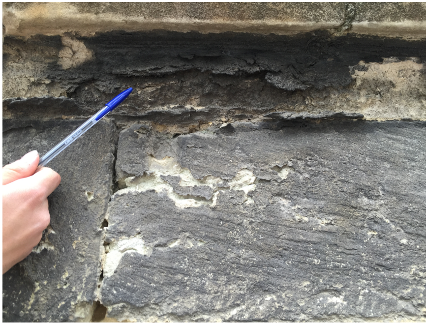
Fig. 1 Thin layer of black crusts formed on a carbonate building stone, on a church wall in Fécamp city.
