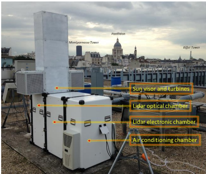
Figure 1: LAASURS system on the Paris Sorbonne University rooftop
