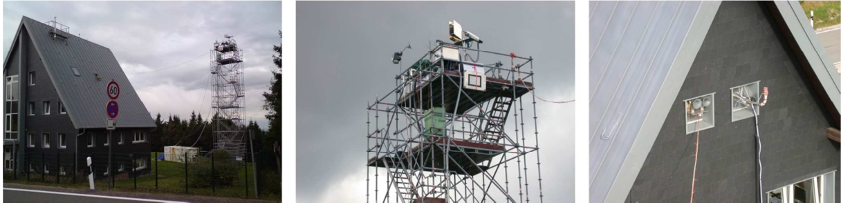
Figure S1: Photographs of the summit site. Left: Measurement building and tower; middle: instruments on the 20 m tower; right: CVI and interstitial inlet at ca. 15 m altitude, facing south-west (215°).
