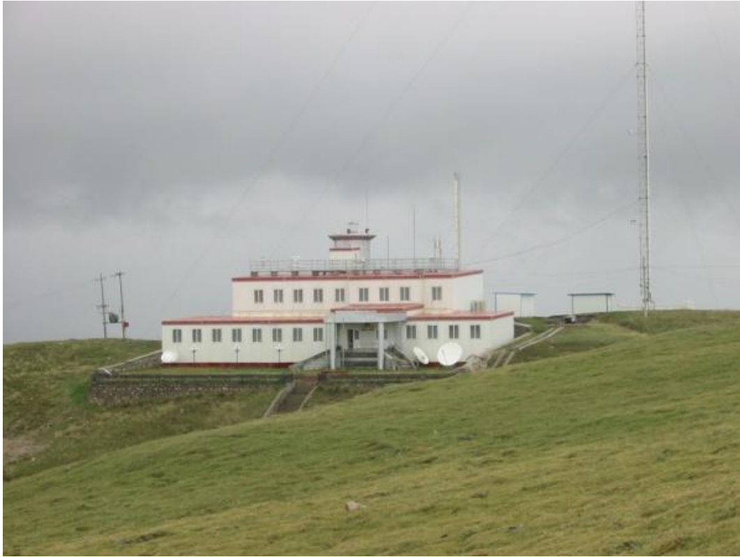
Figure S18: Sampling site Waliguan. Our air sampler was installed on the top of the building (Photo was taken by Yi-Fan Li).
