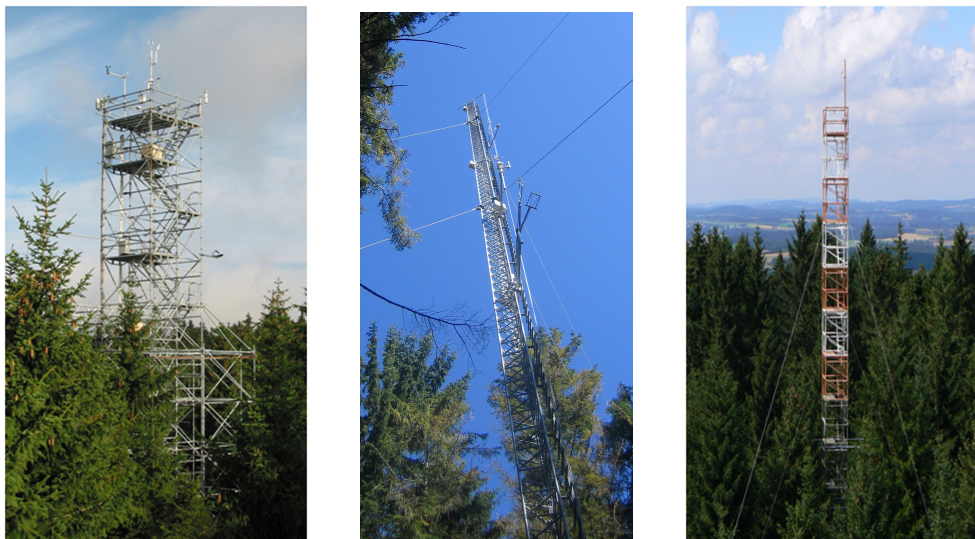
Fig. 6. Towers at the Waldstein-Weidenbrunnen site: (a) permanent main tower since 1996 (height 31 m) for routine measurements, FLUXNET station and chemical measurements, (b) turbulence tower (height 35 m) since 2007 with second FLUXNET complex and turbulence measurements, (c) biological tower (height 36 m) for gas exchange measurements at needles.
