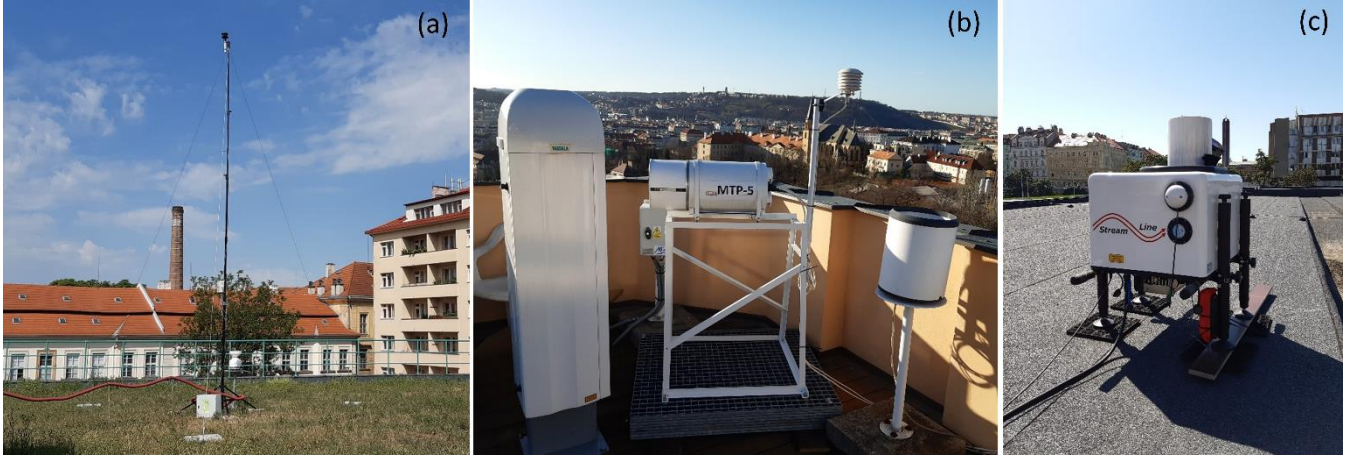
Figure. S4. Supplementary non-reference meteorological measurement used for TURBAN observation campaign: (a) mobile telescopic meteorological mast (MM, height 7.5 m) installed in PVK garden, (b) microwave radiometer MTP-5-He (MWR; for temperature profile measurement up to 1 km height) placed at the Karlov MS; (c) Doppler LIDAR StreamLine XR (for wind and backscatter intensity measurement up to 1.2 km height) placed at the PVK roof.
