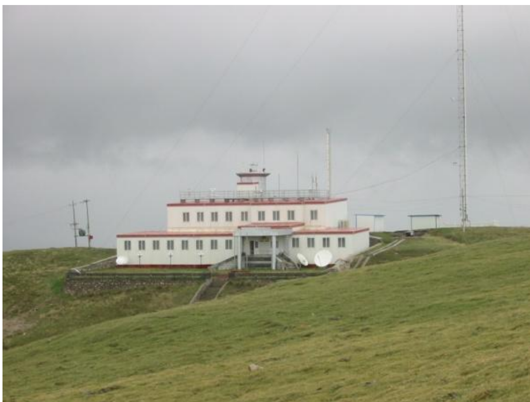
Figure S18: Sampling site Waliguan. Our air sampler was installed on the top of the building (Photo was taken by Yi-Fan Li).
